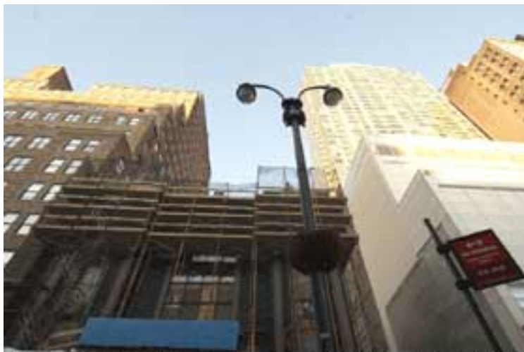
The 1867 Glad Tidings Tabernacle at 325 West 33rd Street is being demolished.
